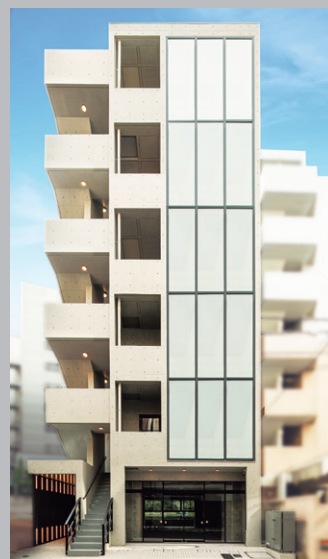
exterior of the building
